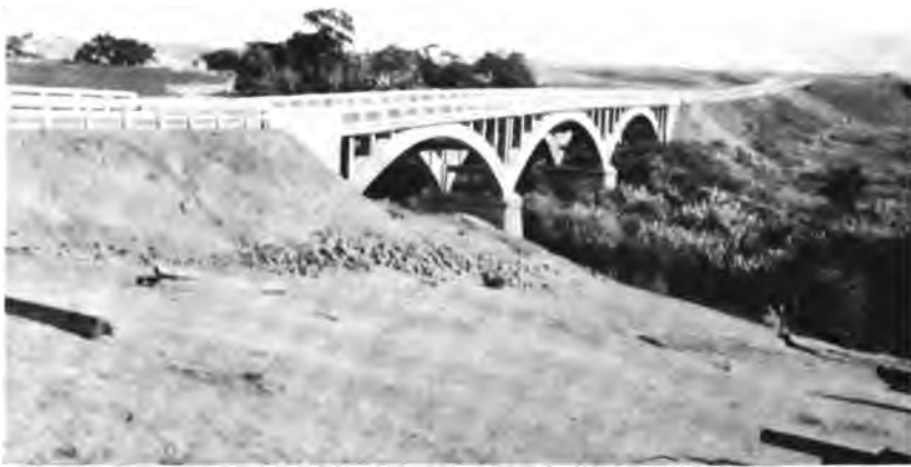
Dry Creek bridge on Stanislaus County highway system.
